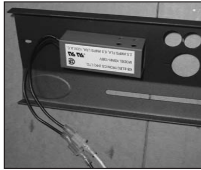
Figure 49. Install Fan Controller.
